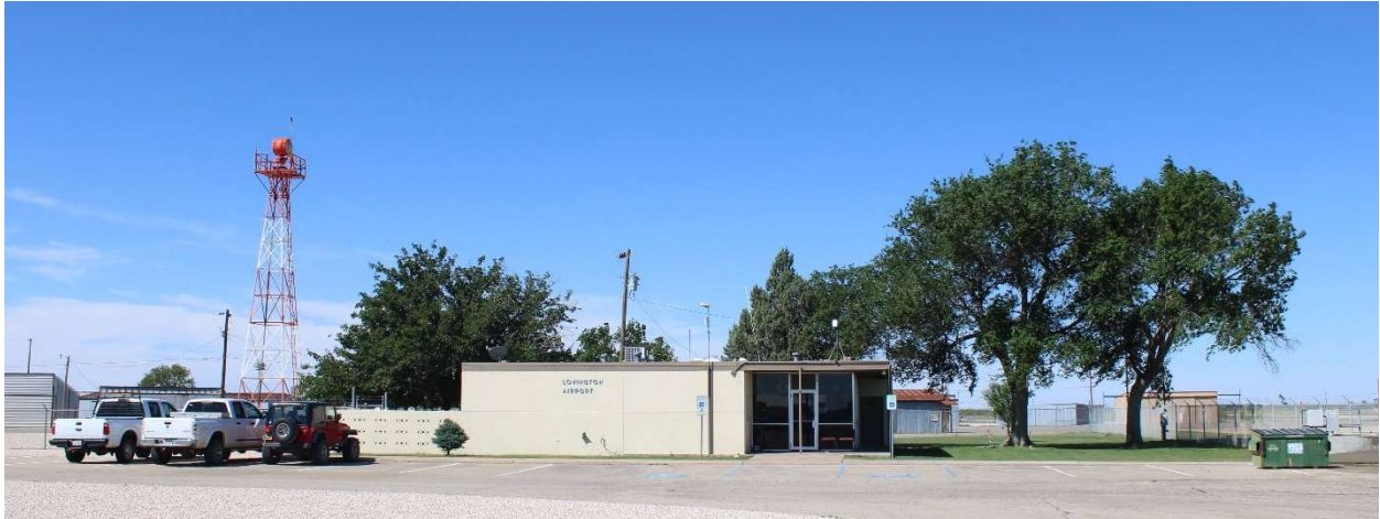
Terminal building at the Lea County-Zip Franklin Memorial Airport.
