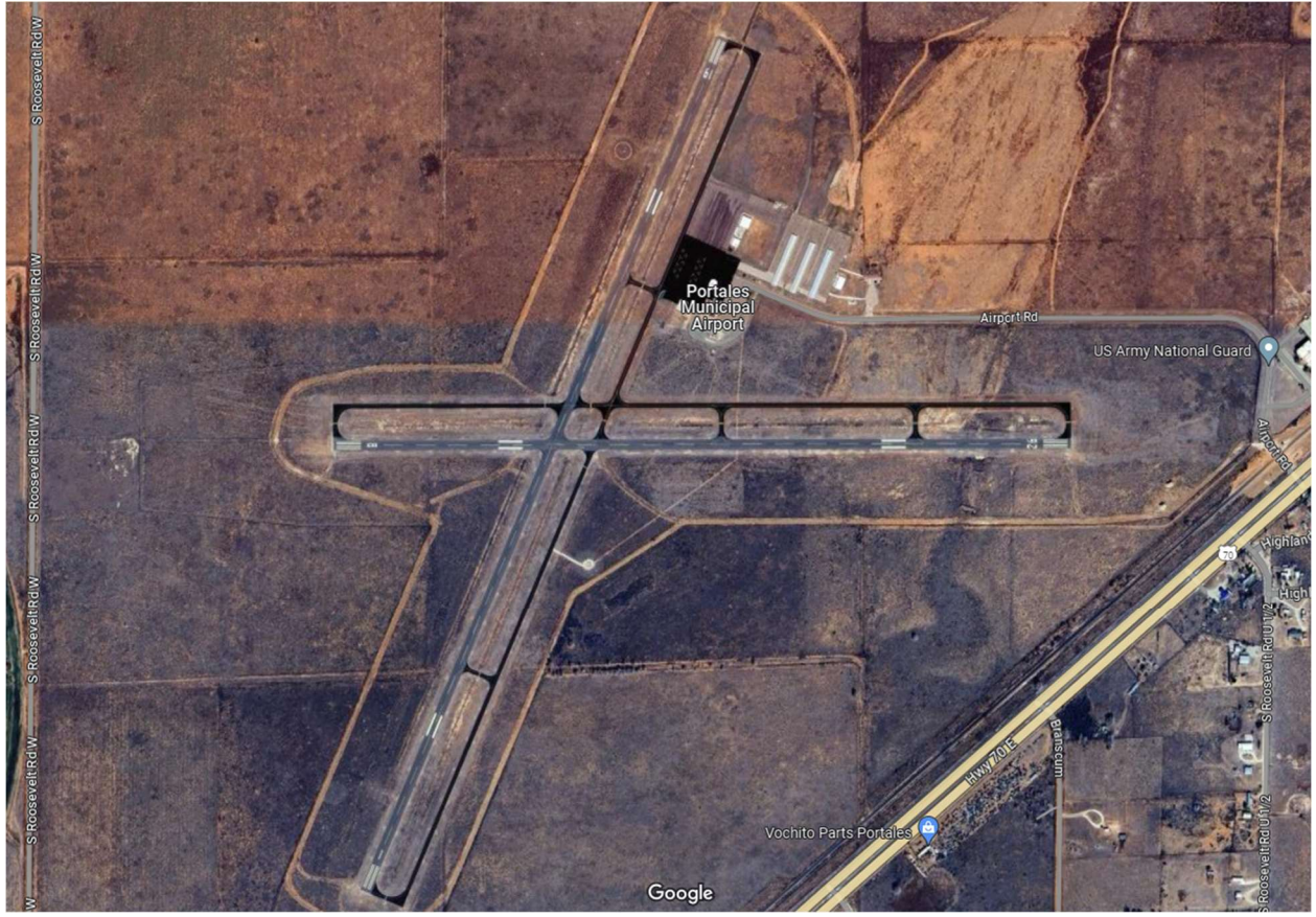
Portales Municipal Airport aerial view.
