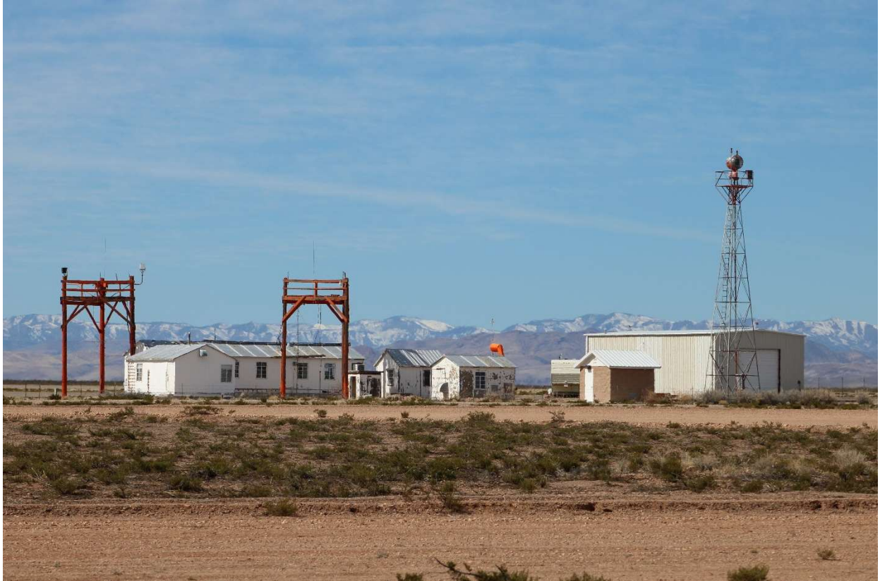
Original 1930's navigational equipment and structures as well as two delta towers still in use at the Truth or Consequences airport.
